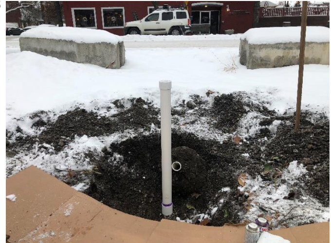
MW-6 PVC casing attached to original well casing.
