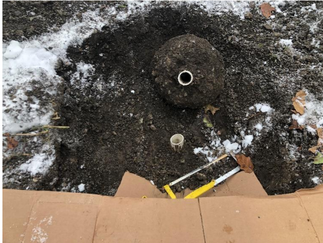
MW-6 casing cut below monument for repair
