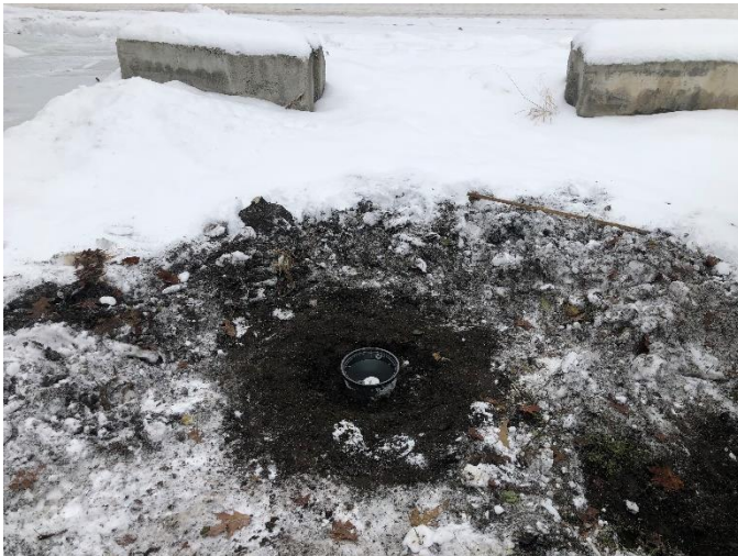
MW-6 PVC cut below grade to fit inside well monument
