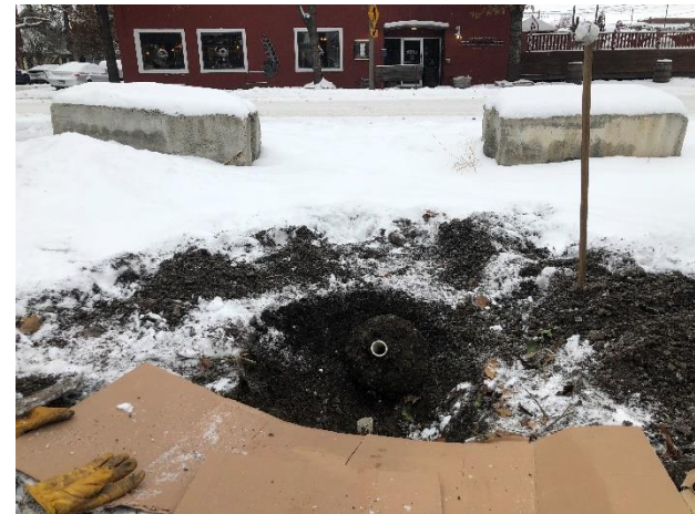
MW-6 casing cut below damaged monument facing north
